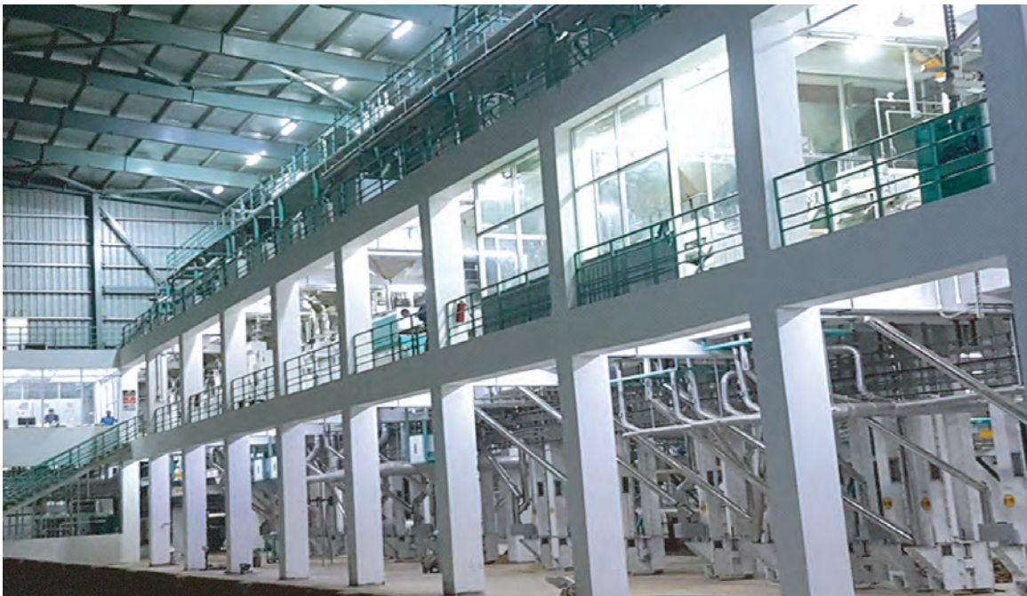
Factory inside View
