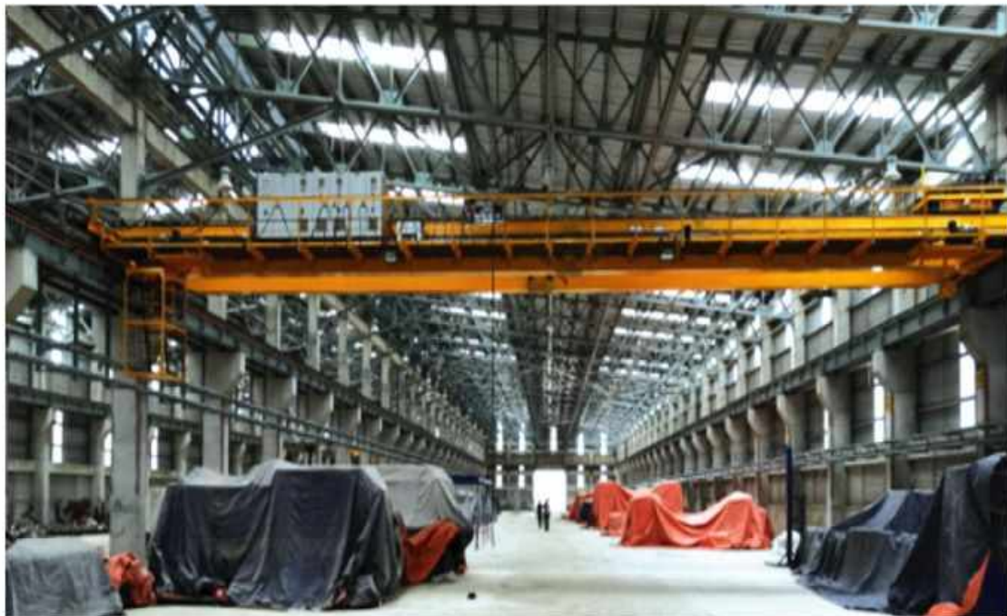
GI Finished Product Shed (under construction)
