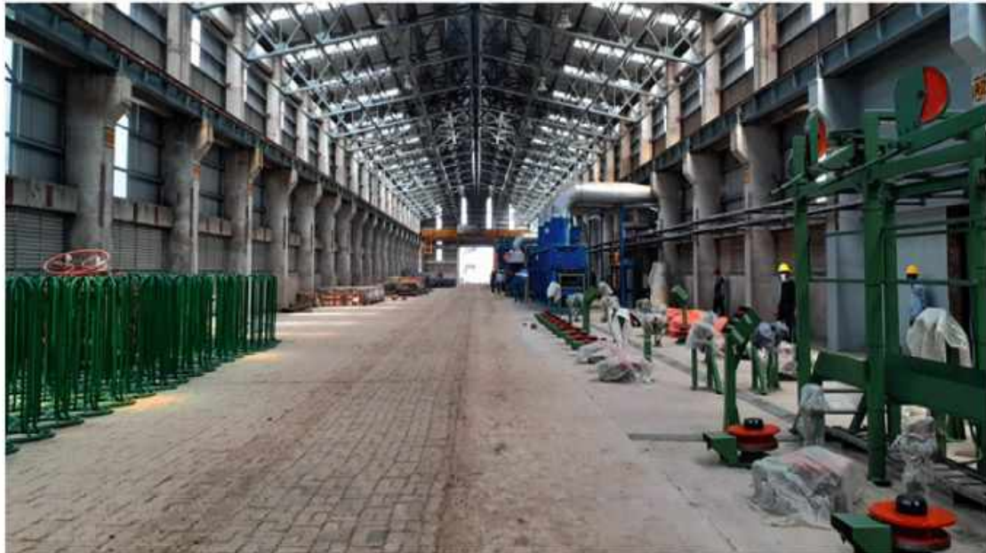
Galvanizing Shed (under construction)
