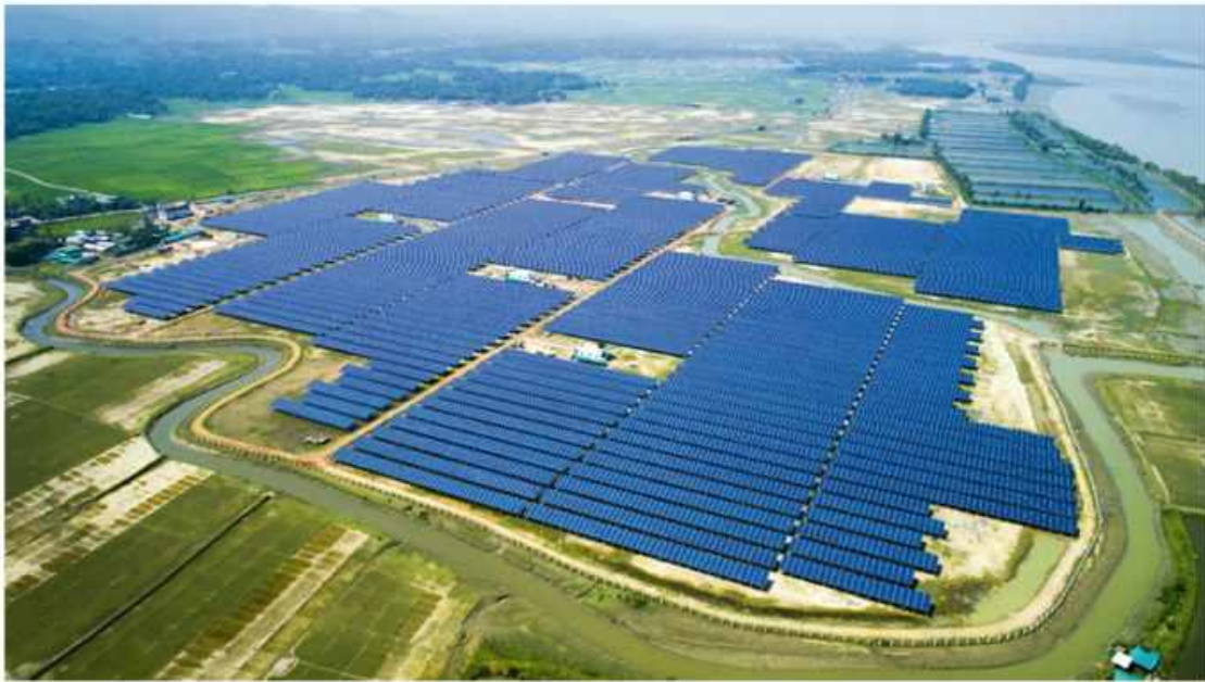
Top view: Solar Power Plant
