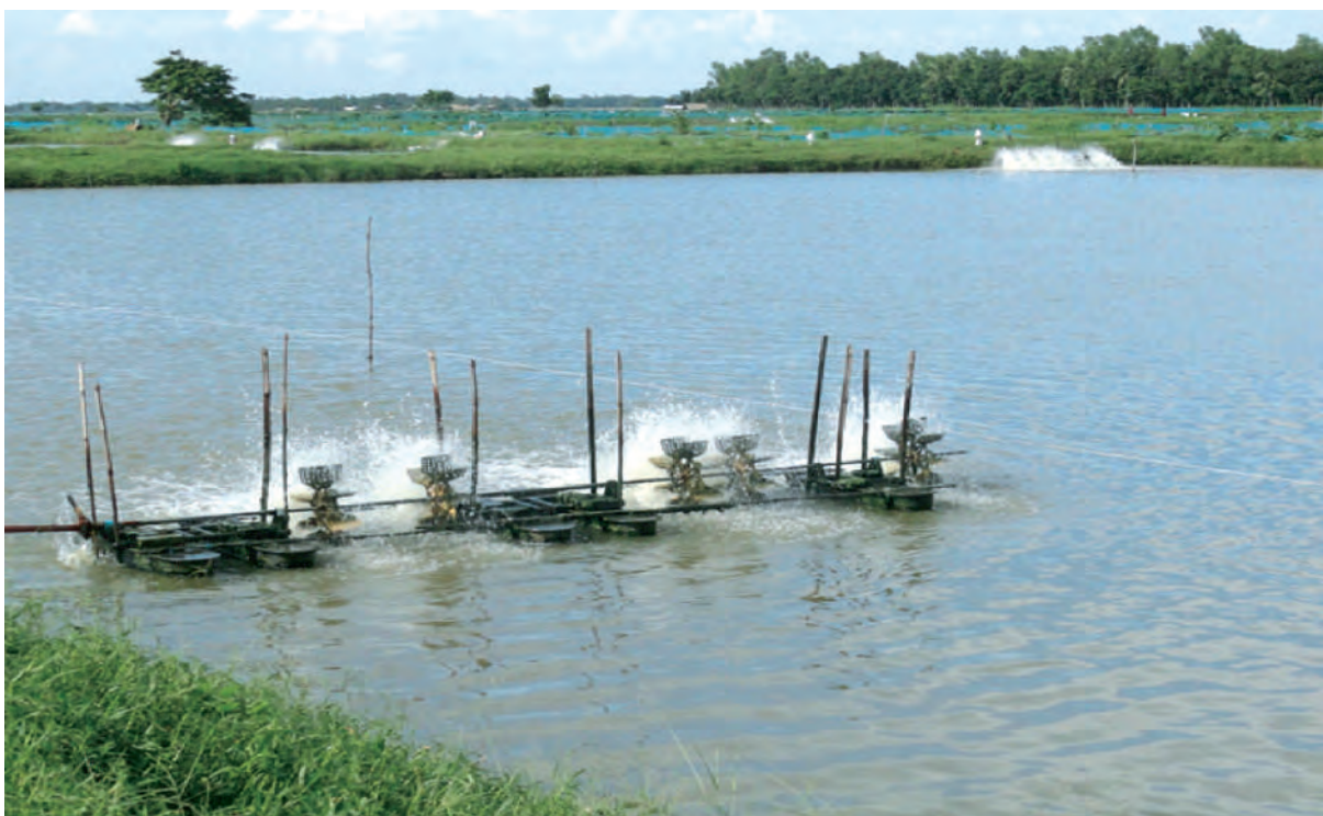
Aeration with Aerators
