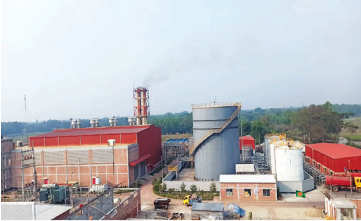
Outside View: Power Generation Plant
