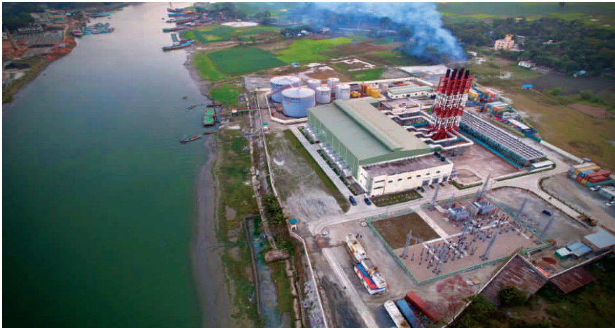
Top View: Power Generation Plant
