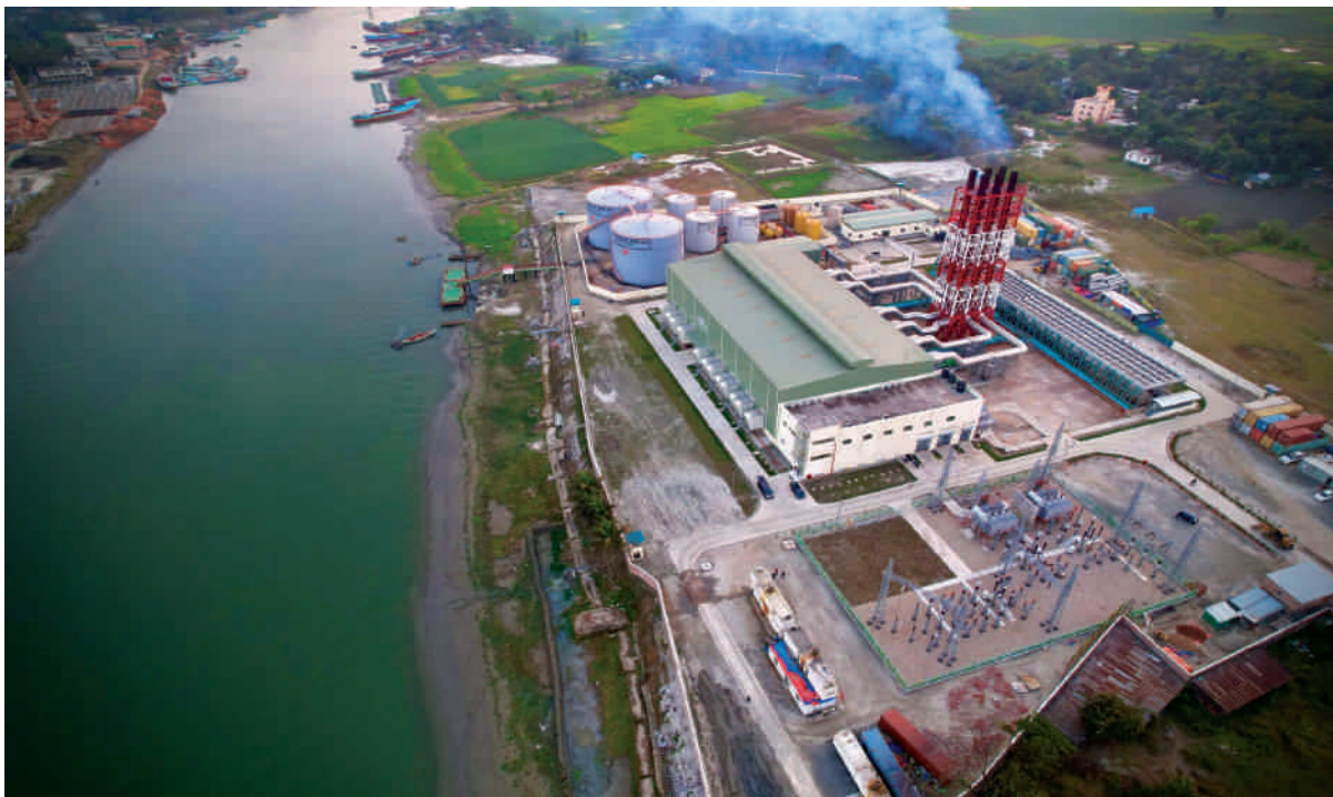
Top View: Power Generation Plant
