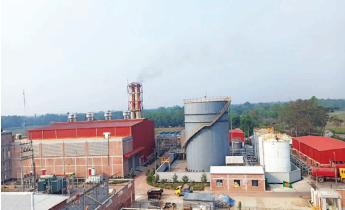
Outside View: Power Generation Plant
